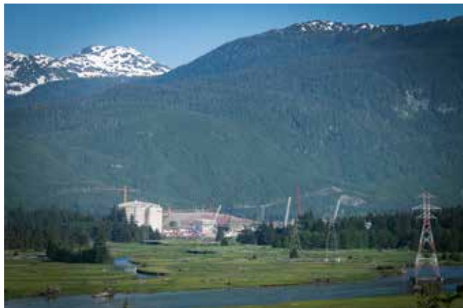
◀ Across the Kitimat River is LNG Canada's natural gas storage tank, which will be one of the largest in the world, at 225,000 cubic metres
