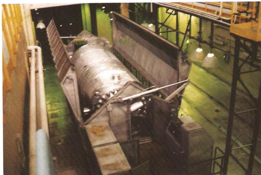
A nuclear waste rail car is unloaded at the Krasnoyarsk facility.
