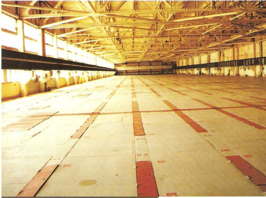
2001: Inside the half-built reprocessing center at Krasnoyarsk.
